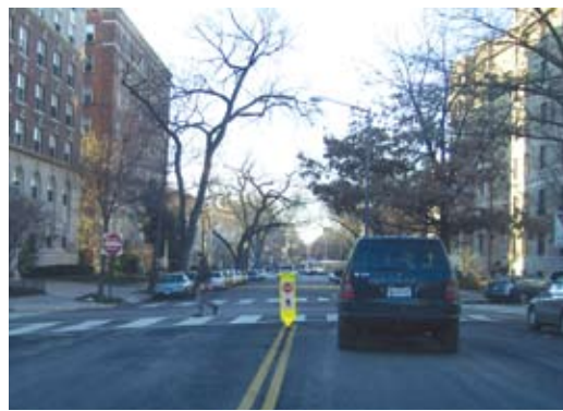
High-visibility crosswalks can be supplemented by “in-roadway pedestrian crossing signs” that remind drivers of state laws requiring them to yield or stop for pedestrians in the crosswalk. Pictured is a ladder type crosswalk marking, with an in-roadway pedestrian crossing sign.
