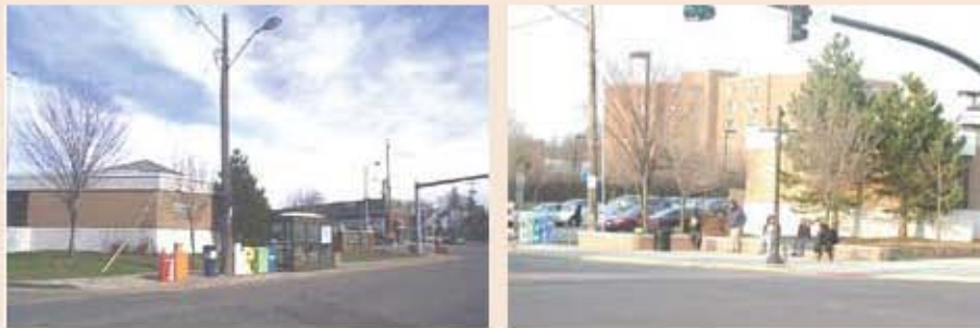
Chagrin Blvd and Lee Road in Shaker Heights, Ohio before (left) and after (right) implementation of the Transit Waiting Environments program. Improvements included: formal and informal seating, more visible crosswalks, wider sidewalks, ADA compliant curb ramps and removal of clutter.
