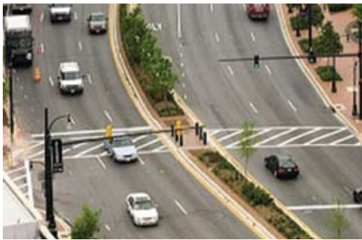
This midblock crossing in Silver Spring, Maryland uses multiple engineering strategies, including pedestrian-activated signals and a median refuge area, to improve safety for pedestrians crossing the street at this busy, urban location.
