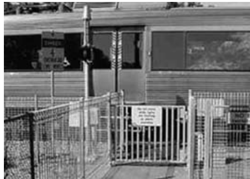
Multiple safety treatments are used at this pedestrian at-grade railroad crossing, including fencing, and warning signs.
