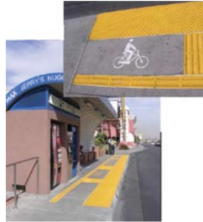
Bus stops may benefit by having separated marked areas for bicyclists to wait for the bus.
