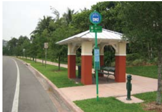
This bus stop includes an attractive pole with route and schedule information. It also includes a shelter, bench, trash can, bicycle rack, and has excellent access to the local sidewalk network.
