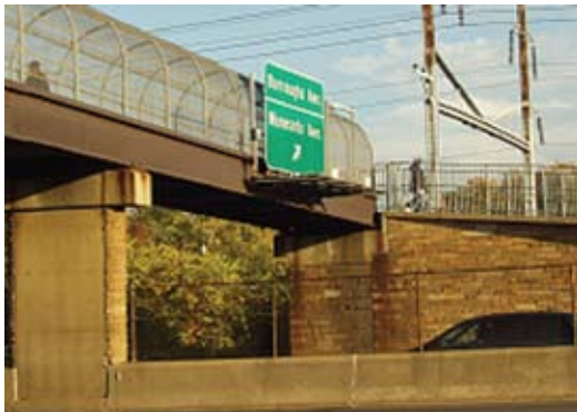
This grade-separated crossing over a freeway allows pedestrians to cross from their neighborhood to a nearby transit station.
