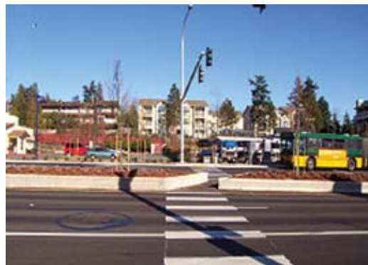
The median island near this transit stop includes an angled cut-through for pedestrians. This feature encourages pedestrians to face to the right and look for oncoming traffic before crossing.
