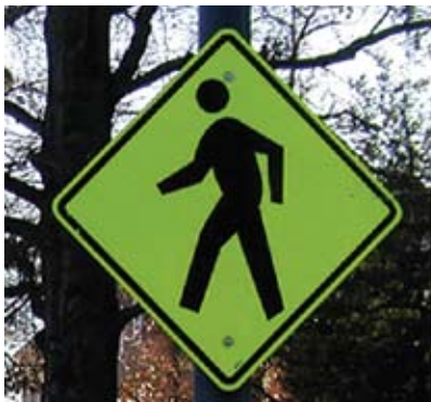
Fluorescent yellow-green pedestrian warning signs can increase driver awareness of pedestrians crossing the road near transit stops.
