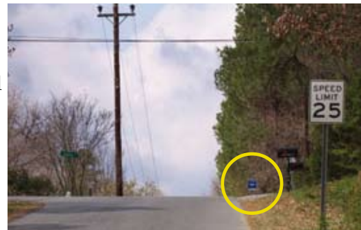
Pedestrians crossing the street to reach the bus stop circled in the photograph above will be hidden by the crest of the vertical curve.
