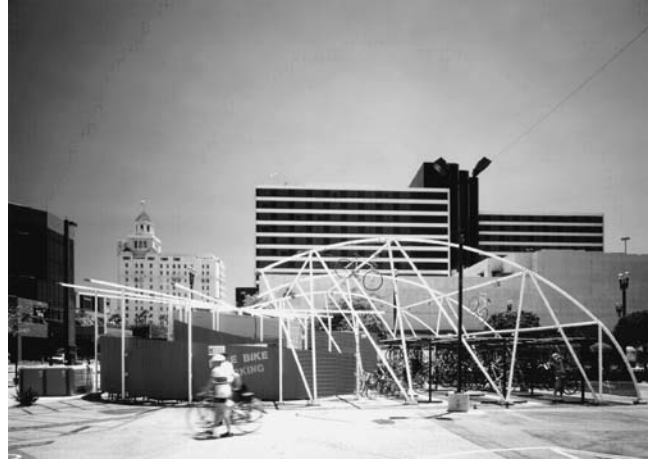
FIGURE 35 New bike station under construction for Bikestation Long Beach.
