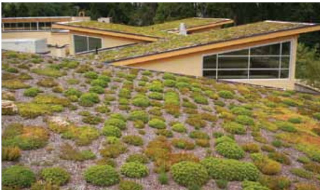
Green Roof at Walter Reed Community Center. Photo by Arlington County, Virginia.
