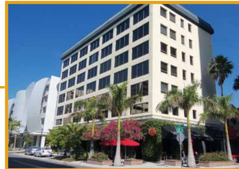
Photo by Jacobs Engineering Group
