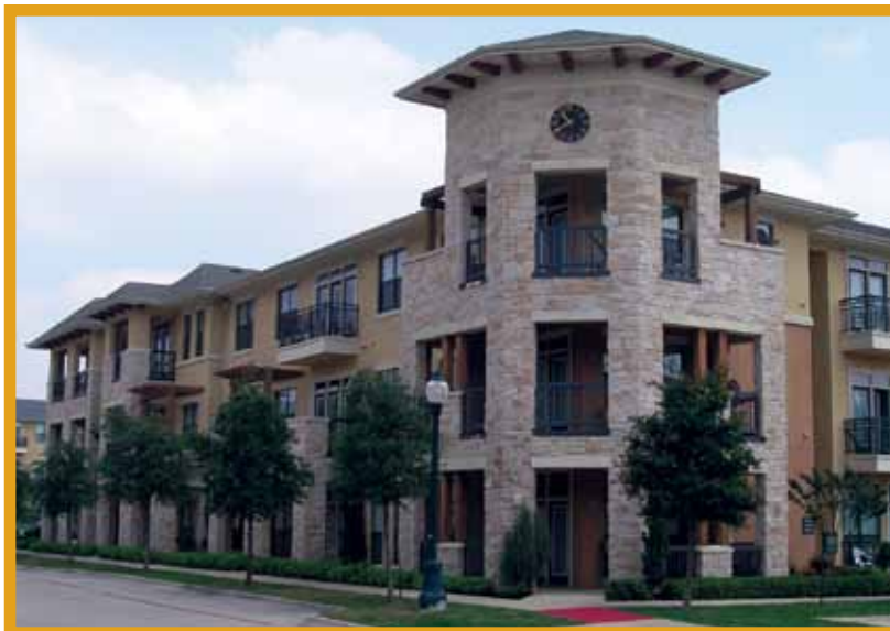
Photo by Jacobs Engineering Group
