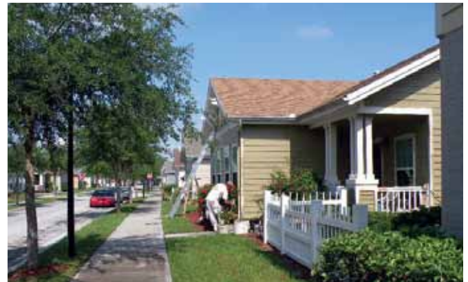
Belmont Heights in Tampa, Florida. Photo by Tampa Housing Authority.
