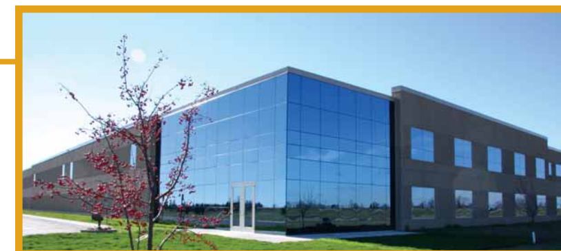
Photo by Jacobs Engineering Group
