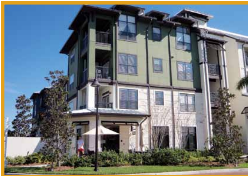
Photo by Jacobs Engineering Group
