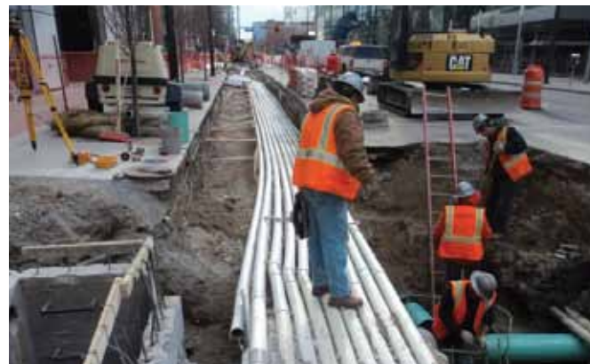
Utility relocation for FasTracks in Denver, Colorado. Photo by Goodbee and Associates.
