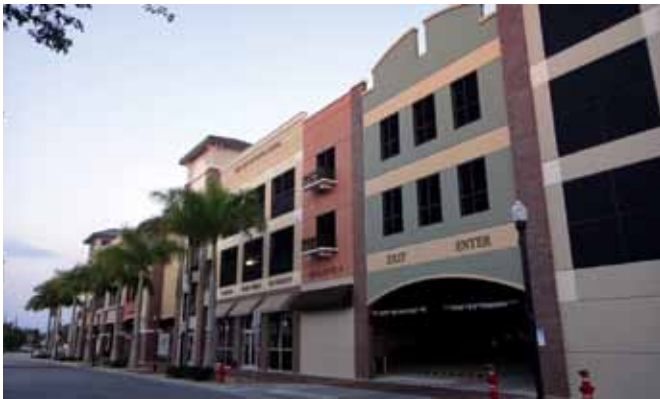
Punta Gorda, Florida. Photo by Jacobs Engineering Group.
