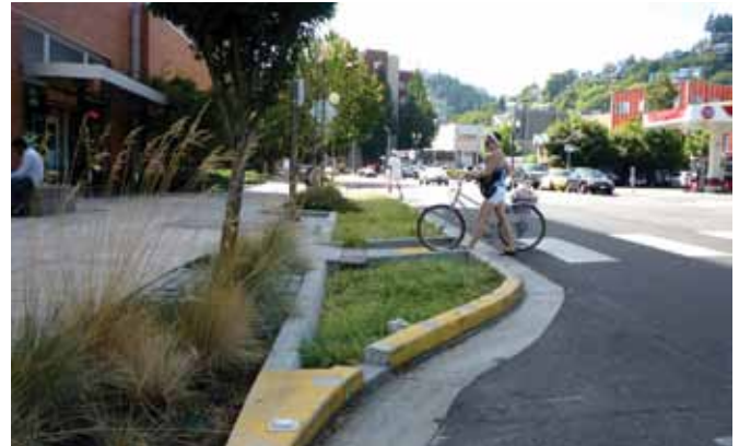
Example of a bulb out. Photo by City of Hoboken, New Jersey.
