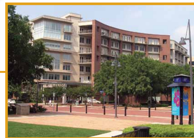
Photo by Jacobs Engineering Group
