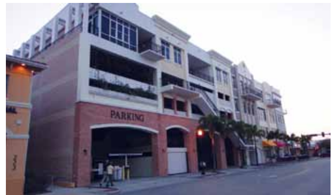
Parking Garage in Punta Gorda, Florida. Photo by Jacobs Engineering Group.
