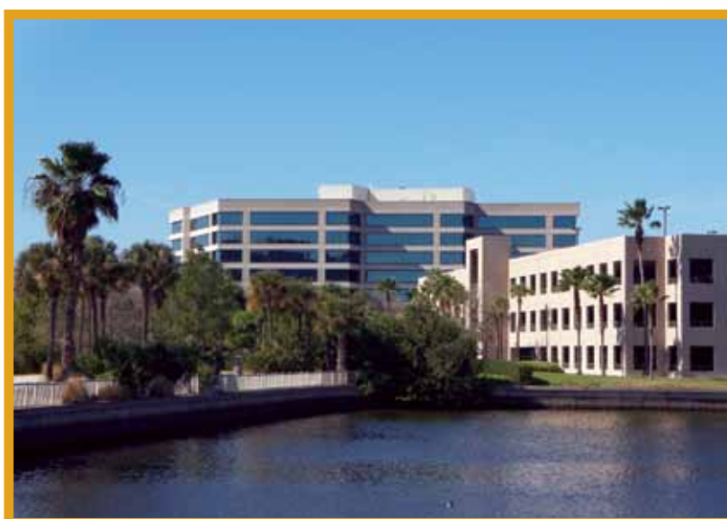
Photo by Jacobs Engineering Group
